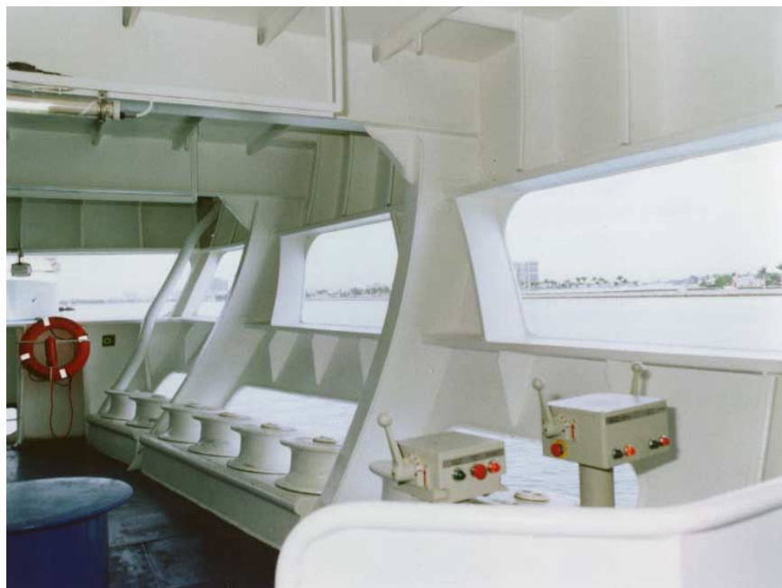
Figure 6b. The Ecstasy's mooring station is a covered deck area that is open to the weather on the side and rear of the ship.
