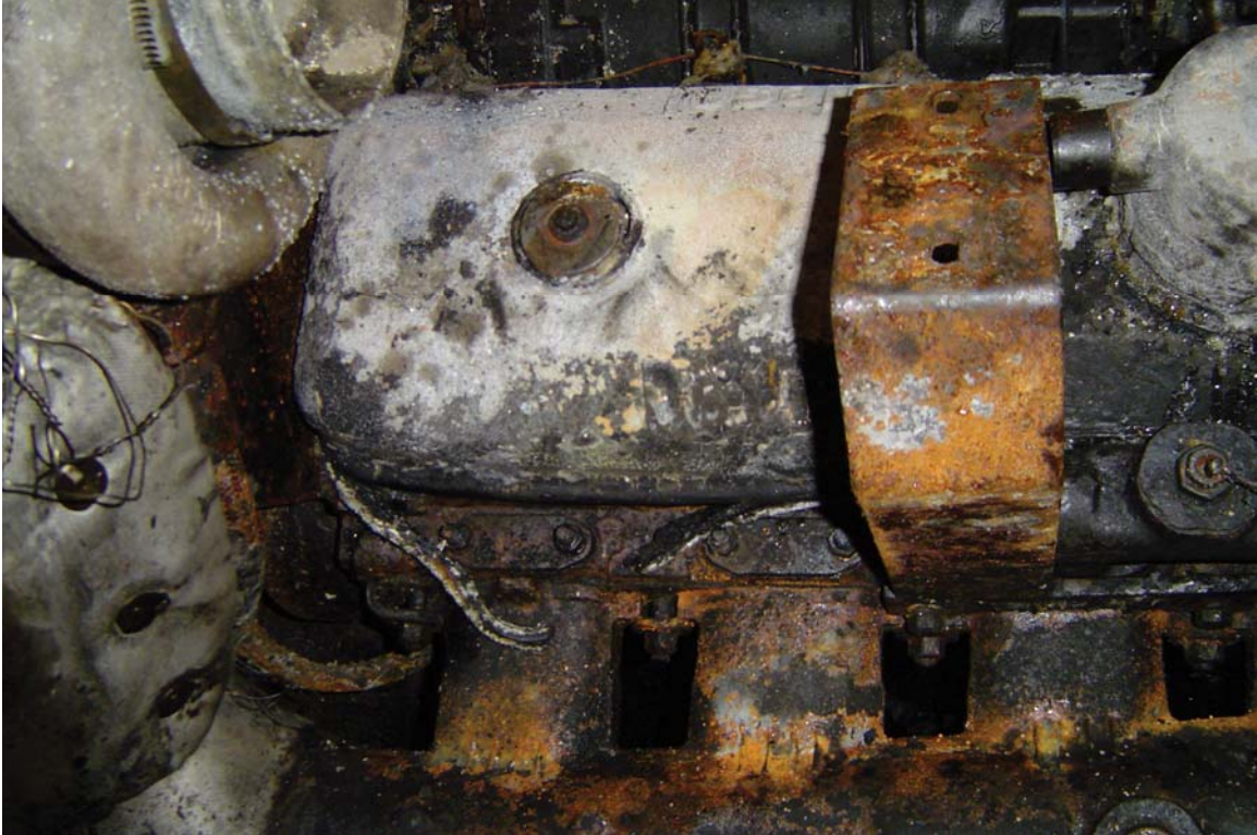
Figure 8. Inboard valve cover and protruding gasket, port inboard engine.
