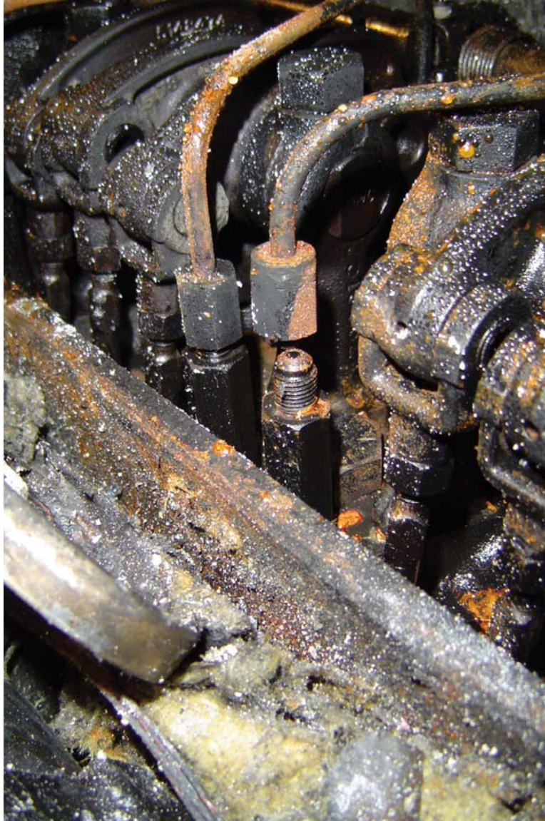
Figure 9. Disconnected fuel line on No. 3 cylinder of port inboard engine.
